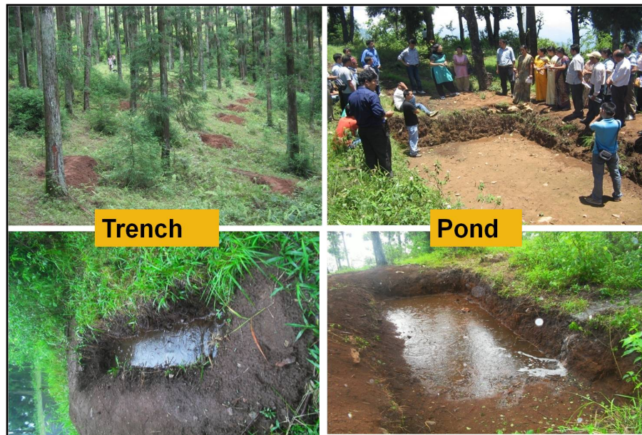
Fig 5: Trenches and ponds trapping the runoff to supplement ground water recharge and enhance the hydrological contribution of mountain ecosystems
