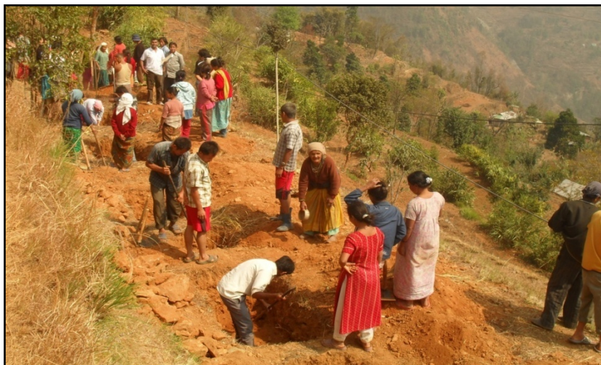
Fig-1: Women taking the lead to construct rainwater harvesting structures in the recharge area of the springs to augment the groundwater
